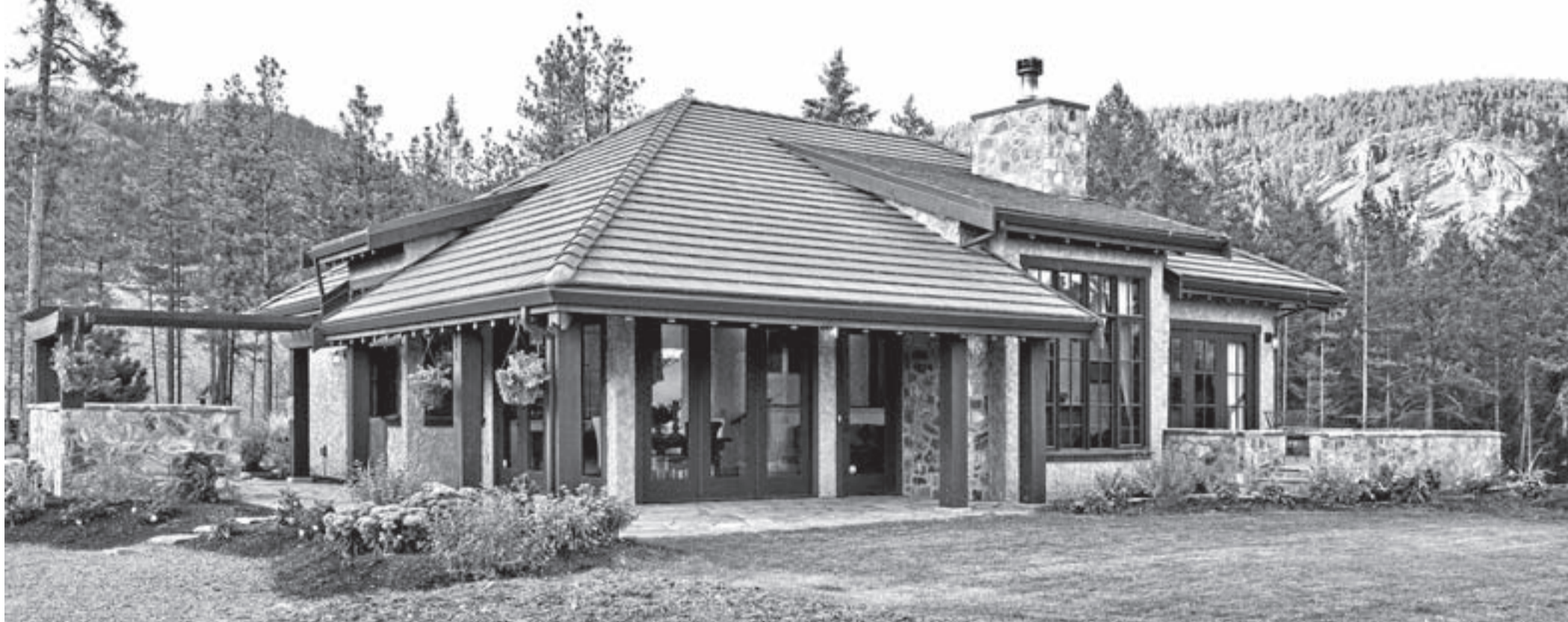
Architect John Sproule envisioned an Old World/New World fusion of styles at Trepanier Manor in Peachland, B.C. The homes feel like a North American take on an English country cottage. SPROULE + ASSOCIATES
